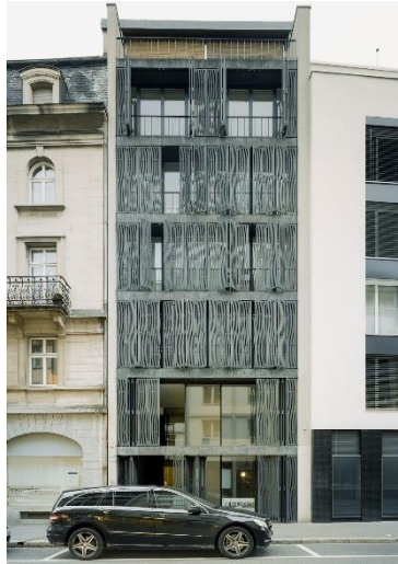
ábra 13 025 Apartment and Commercial Building
