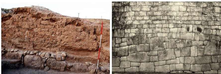
Figure 1: One of the oldest remaining walls in Jericho (left) built around 8500 BCE [1] with patterns similar to brick bonding . Inca wall in Cusco, Peru (right) in which wall bond is not defined yet.
