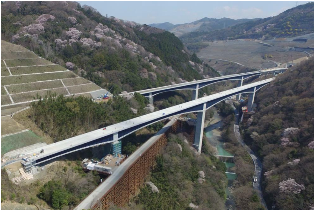
2.10. Figure: Aigawa bridge, Japan [32]
