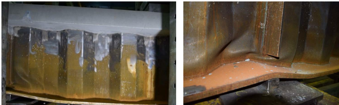
6.4. Figure: B-1-2 Patch loading failure at the support
