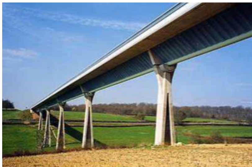
2.7. Figure: Maupre Viaduct, France [29]
