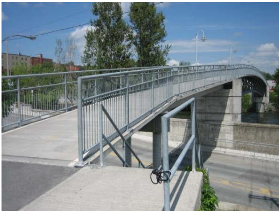
2. ábra: Sherbrooke-Footbridge ( https://structurae.net )
