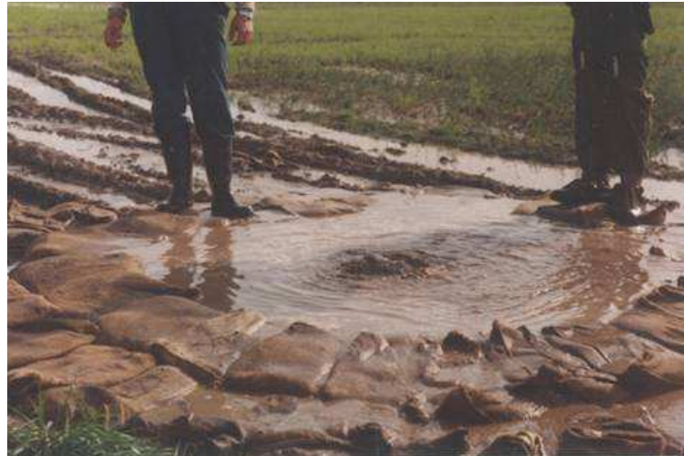
Pic. 12: Jetting near Tiszasas
