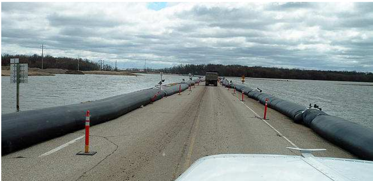
Pic. 24: Well-placed tube dykes along a country road in the US
