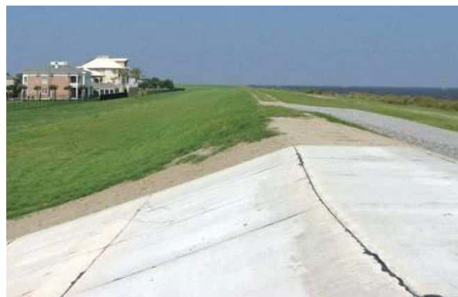
Pic. 39: Concrete, sand and grass in a short section
