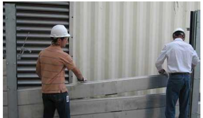
Pic. 21: Installing this kind of wall
