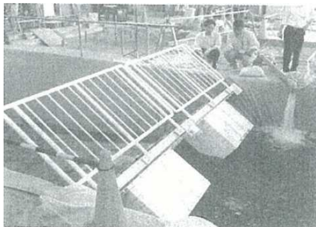
Pic. 32: The water raising the sidewalk and it becomes a flood protection wall
