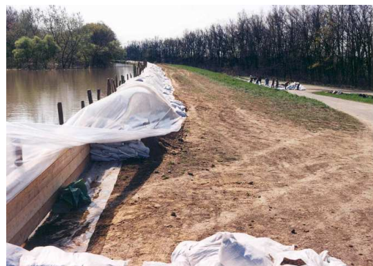
Pic. 16: Waterside boarding under construction at Tiszasüly, 2000
