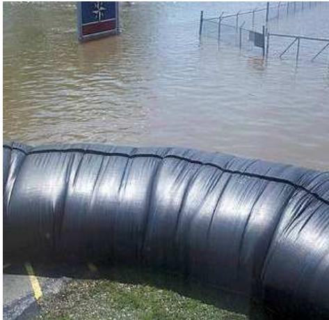
Pic. 22: The nominal diameter (here 1.5 m) is always bigger than the real because of the Poisson-effect
