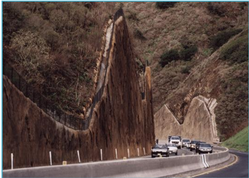
2. ábra: Talajszegedett rézsű, a természetbe illesztve (California Department of Transportation, annual accomplishment report, 2004)
