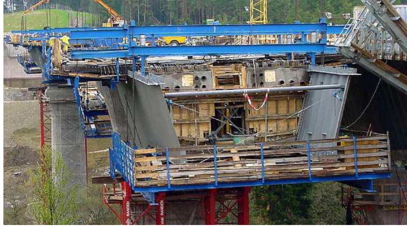
Fig. 10: Corrugated web girders used in bridges, from [39].
