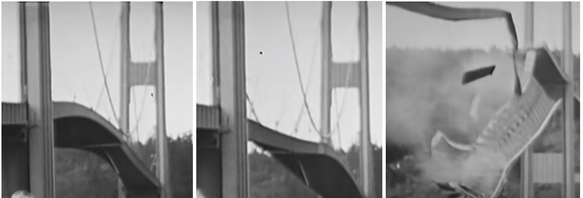
Figure 1.3. Oscillations and the collapse of Tacoma Narrows bridge [17]
