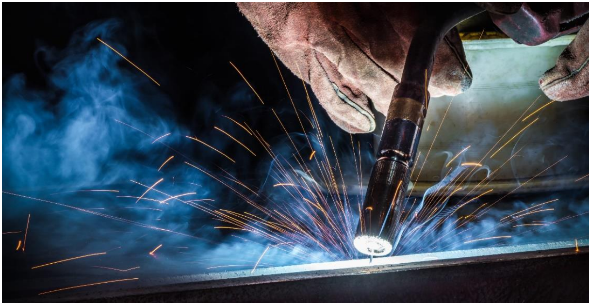
Fig. 7 - MIG/MAG welding during manufacturing [3]
