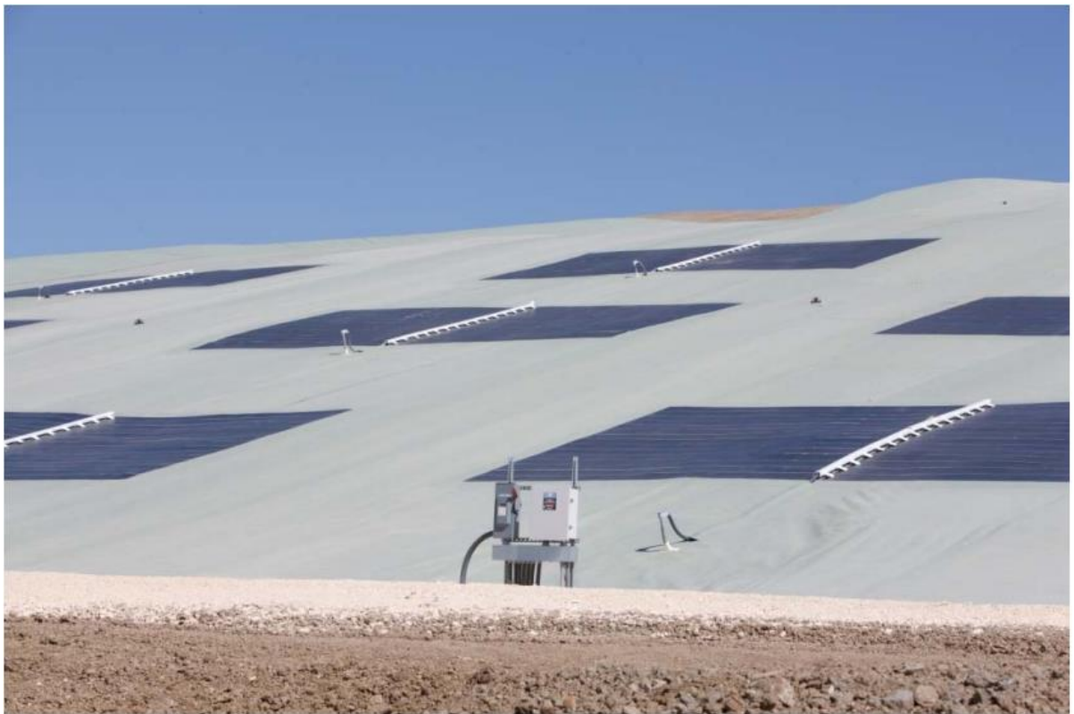
7. ábra. Geomembrán (flexibilis) PV a Tessman Road-i hulladéklerakón Texasban (SAMPSON G, 2009)
