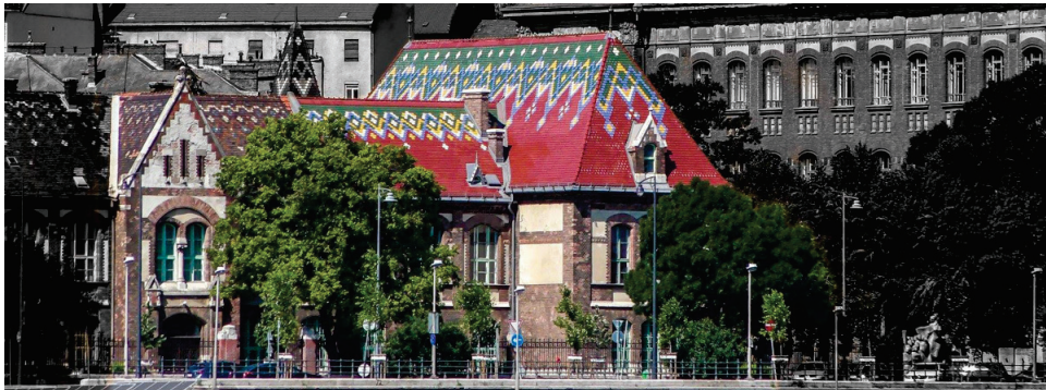
Figure 5.3: Building of Department of Applied Mechanics [3]
