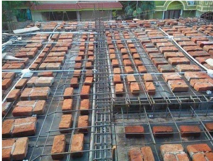
Figure 11: Brick Slab with reinforcement[17]
