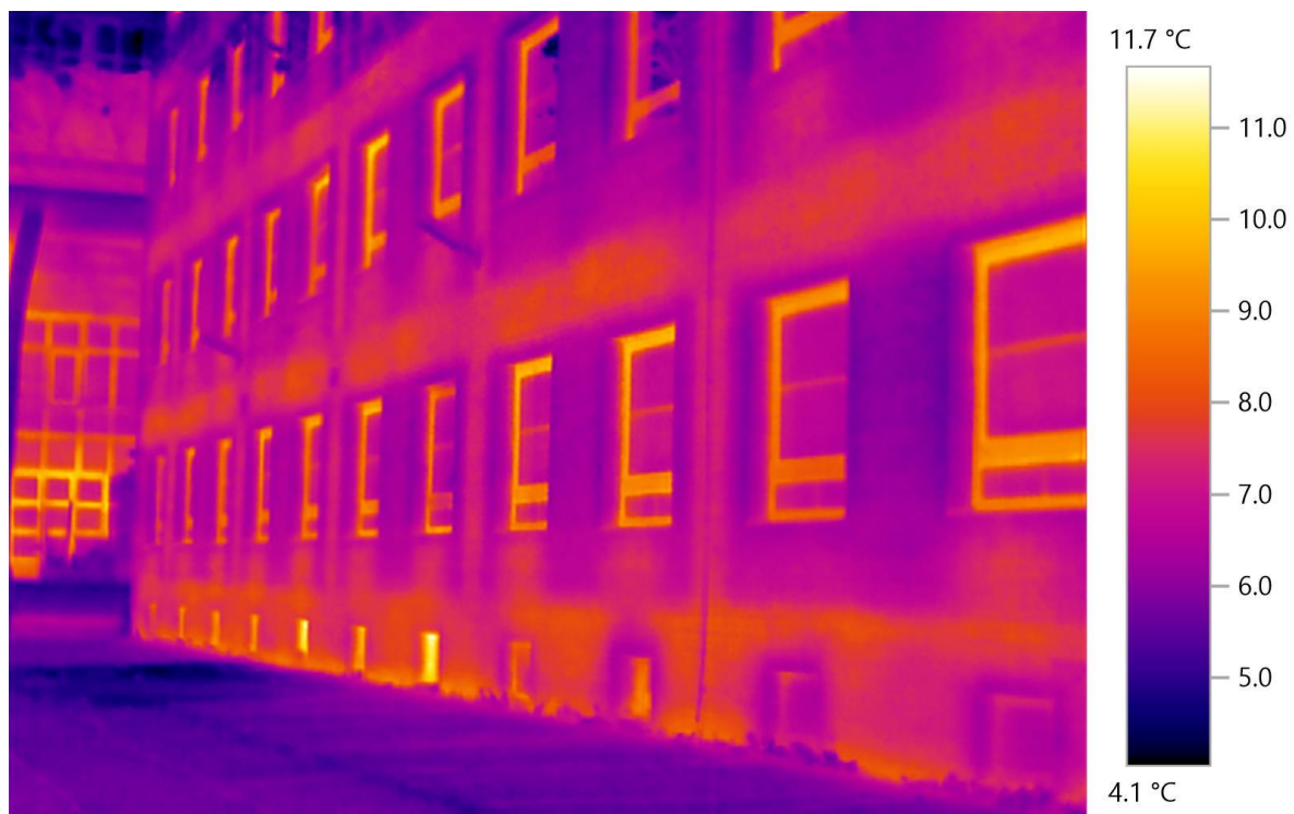
Figure 12 Thermal bridges and structure on the envelope
