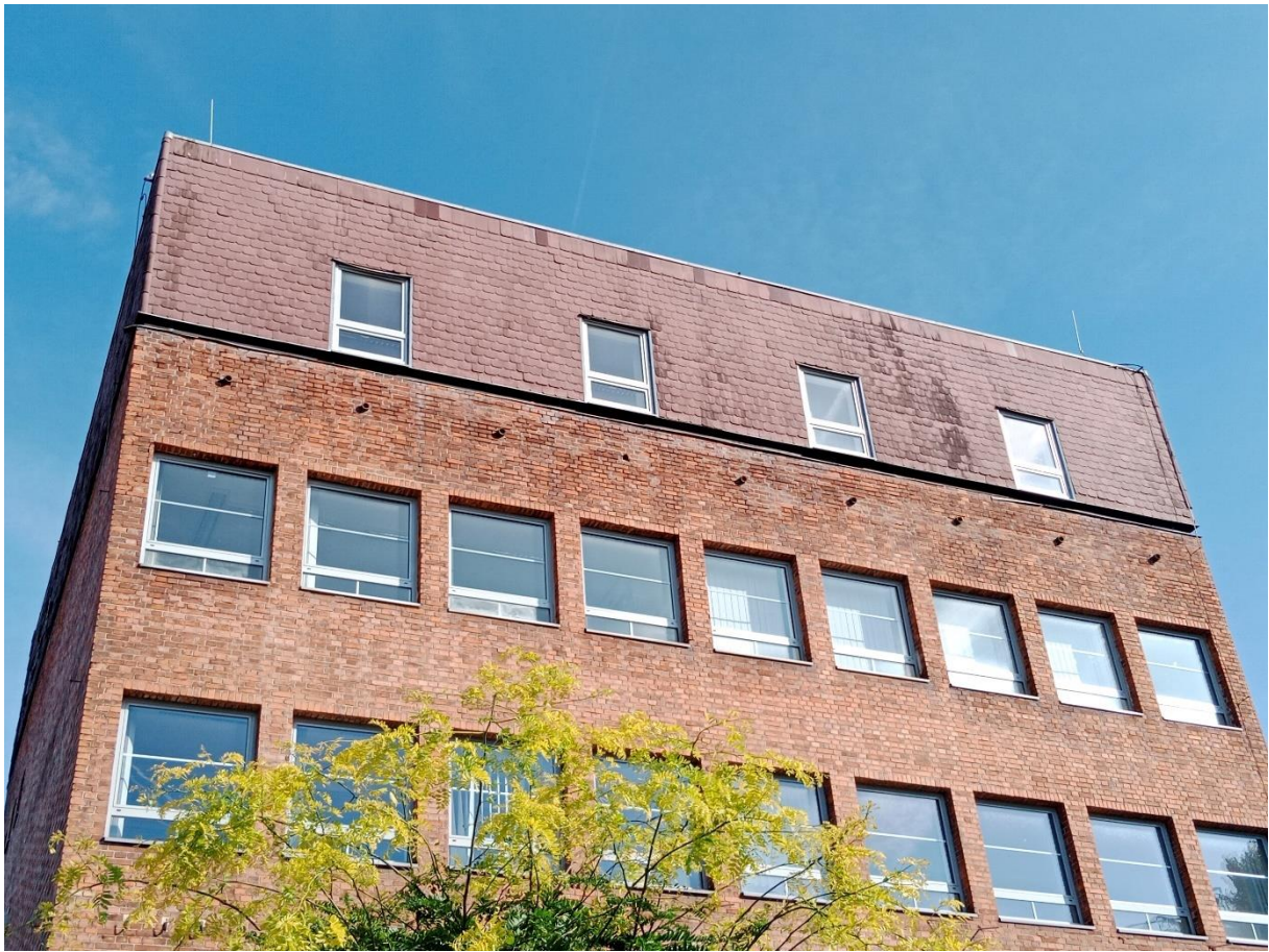
Figure 8 Air vent holes on the facade
