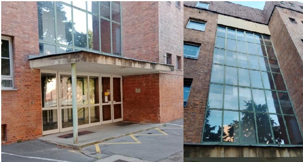
Figure 6 the secondary entrance and the curtainwall in different perspectives
