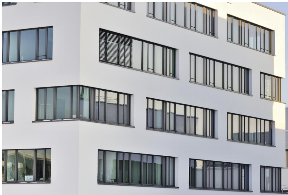
Figure 31 SCHÜCO AWS 75.SI window system [58]
