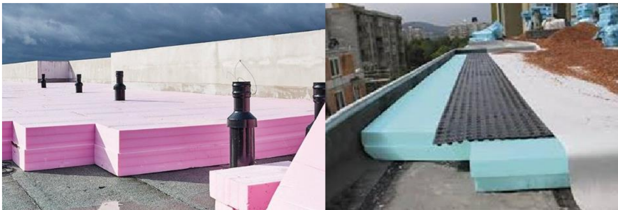
Figure 23 XPS roof insulation [25] [46]
