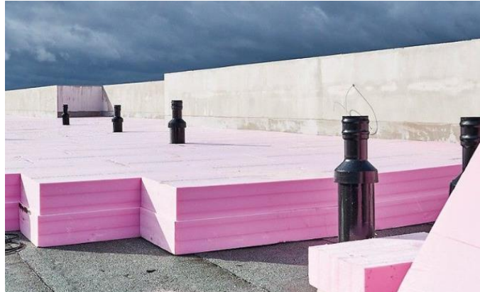
figure 7 XPS roof insulation while installation [23]
