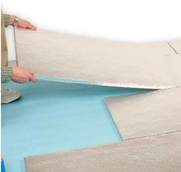
Figure 10 VIPs being installed [87]
