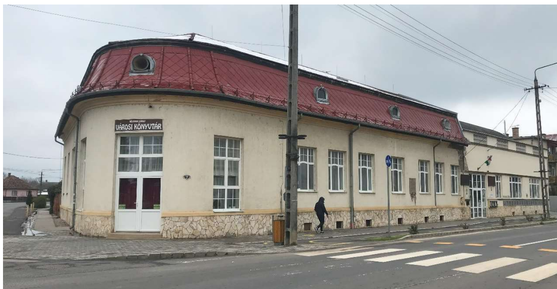
Figure 10. Former Jewish House, currently operating as the Local Library and House of Culture Source: Author, 2023
