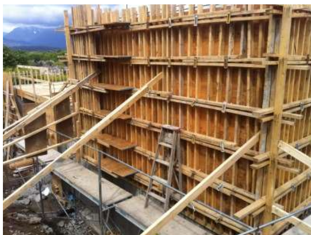
Figure 3. Wooden Formwork in Construction in Medan (source: PT. Sinartech Beton Perkasa [20])
