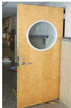
Figure A5. Wooden Interior Door at Sandy Hook Elementary School (Bates)
