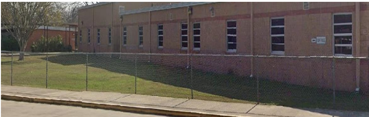
Figure C3. Perimeter Fence at Robb Elementary School (Kilander, Gustaf, and Abe Asher)
