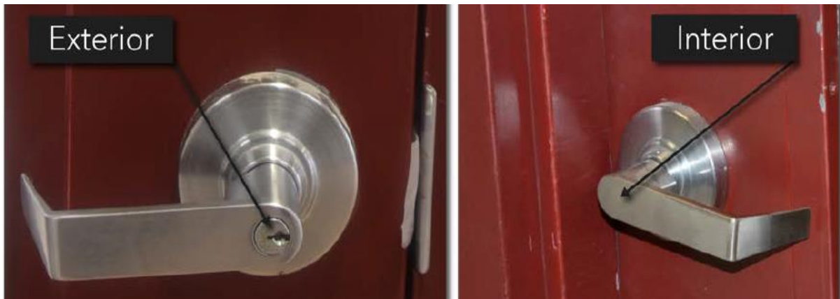
Figure B7. Interior Door Lock of Building 12 at Marjory Stoneman Douglas High School ( Marjory Stoneman Douglas 45 )
