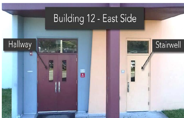
Figure B5. Exterior Doors of Building 12 at Marjory Stoneman Douglas High School ( Marjory Stoneman Douglas 44 )
