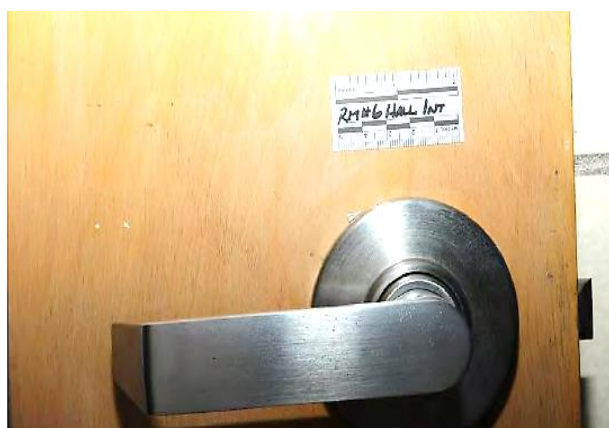
Figure A6. Interior Door Lock (Classroom Side) (Appendix to Report A178)
