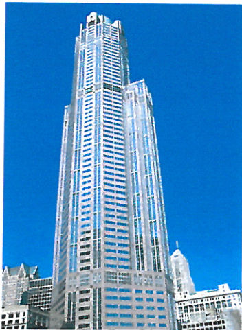
Figure 1: South Wacker Drive 311
