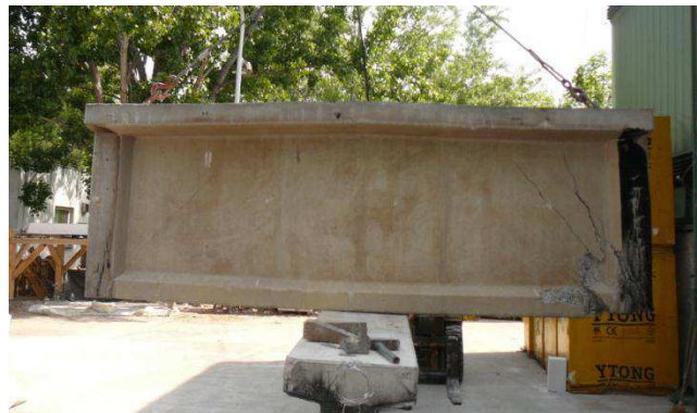
Figure 5: Beam with Mix C after failure in 71 minutes
