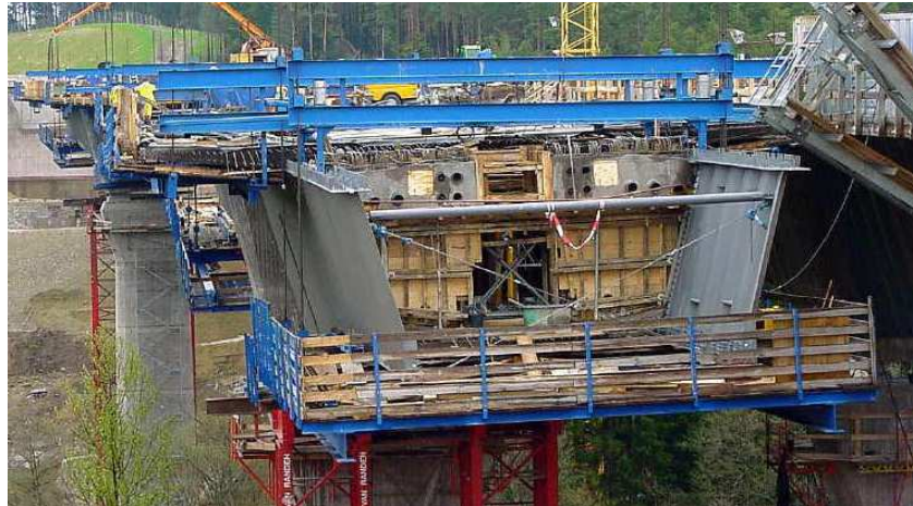
Fig. 7: Corrugated web girders used in bridges, from [39].
