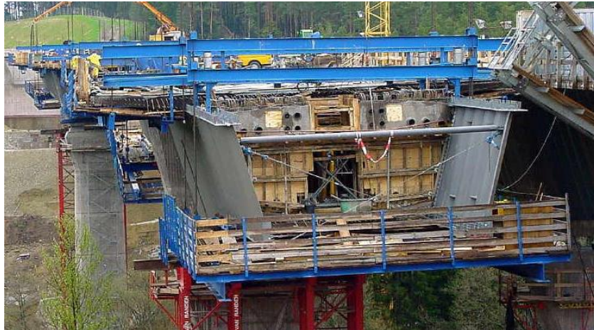
Fig. 7: Corrugated web girders used in bridges, from [36].
