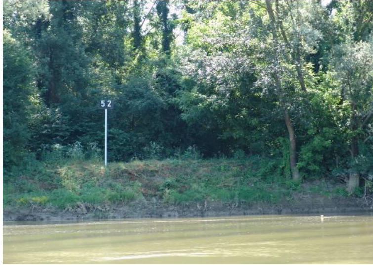
Beginning of the route, existing embankment on the right riverbank
