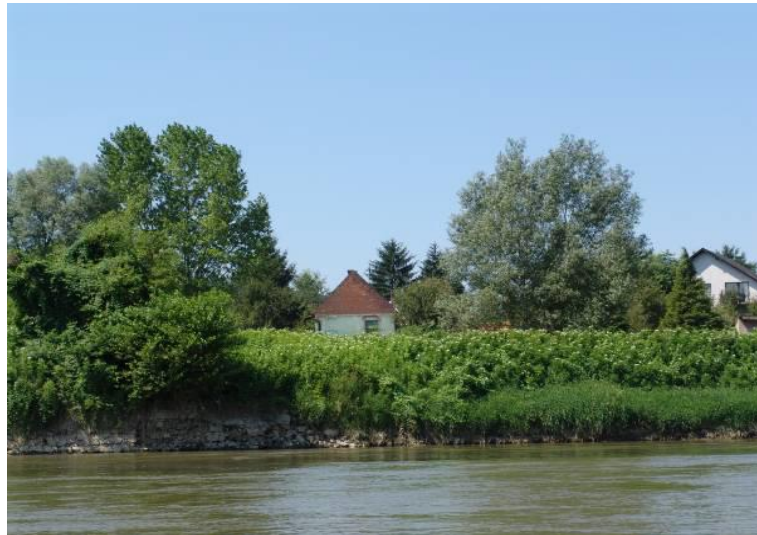
Existing embankment on the right bank, upstream of 52 km
