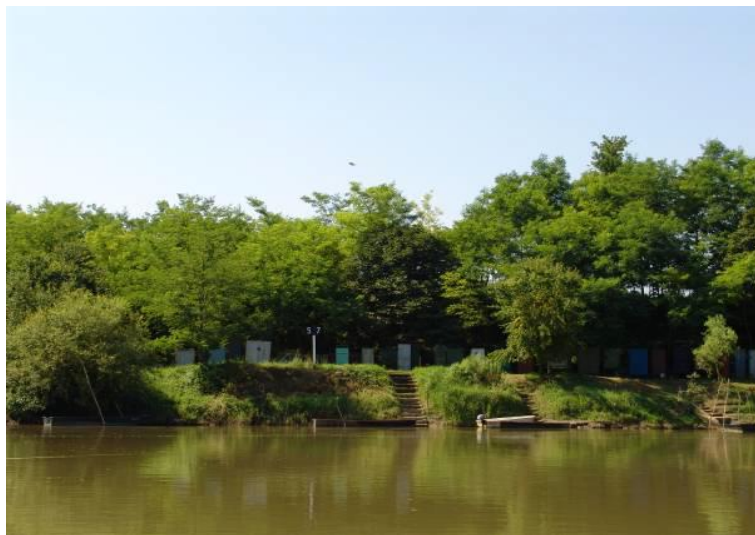
Existing embankment on the right riverbank, 57+000 km
