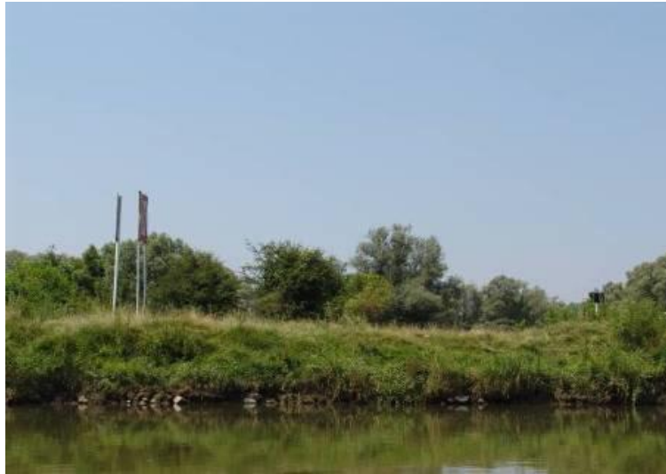
Existing embankment, 70+000 km
