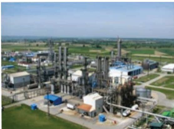
Fig. 3. (a) Gas Processing Facilities Molve (GPFM)
