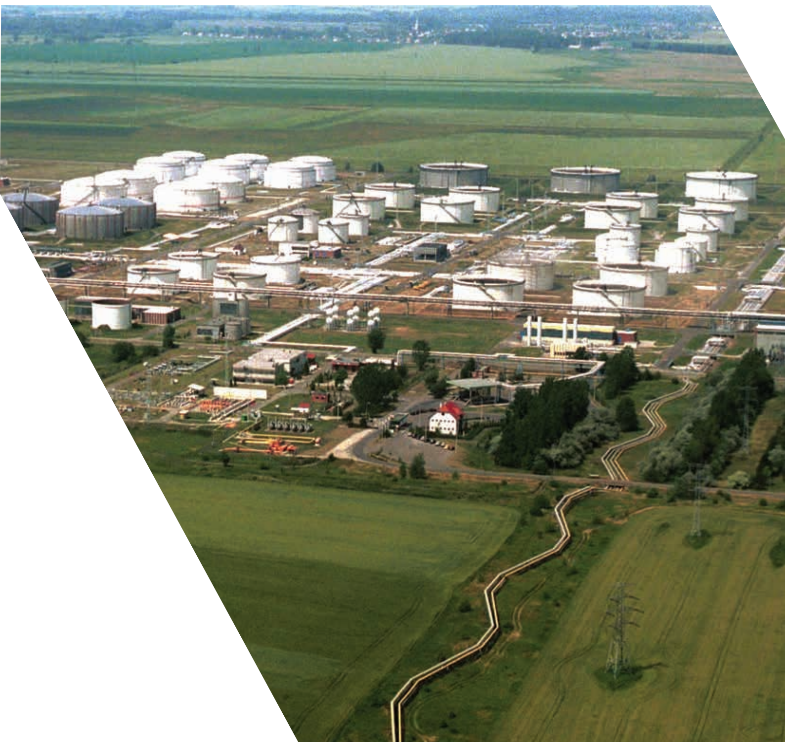
Crude oil storage park
