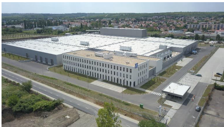
The new plant
