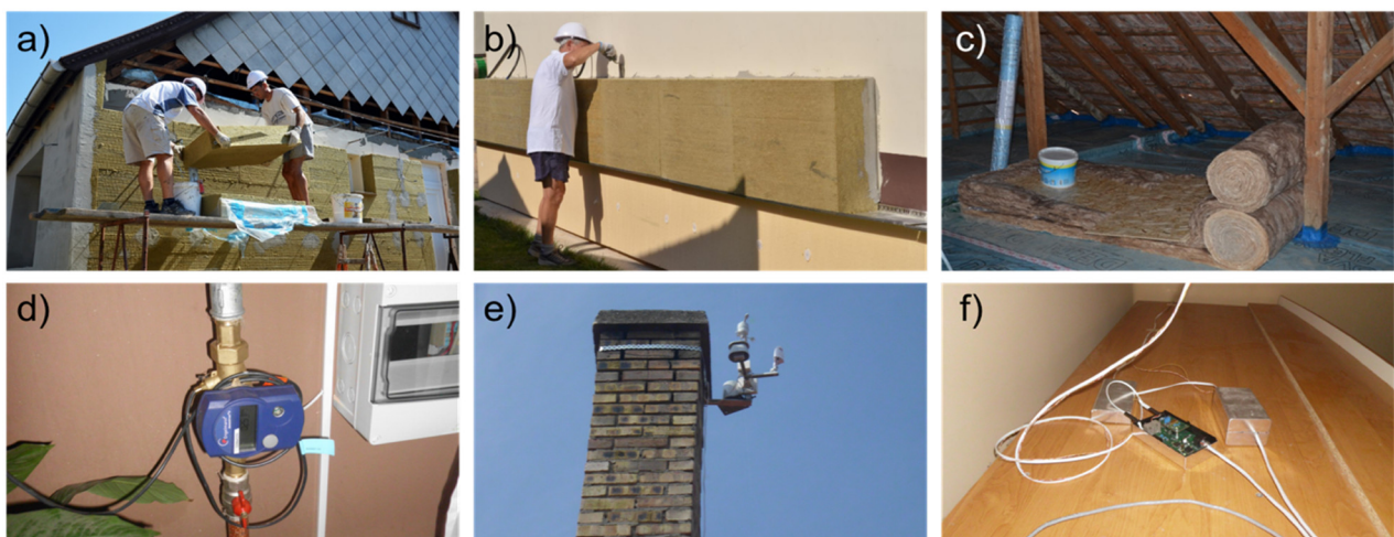
Figure 5: a) and b) wall insulation installation c) attic insulation process d) thermal energy meter built into the heating system e) hygrothermal monitoring system weather station on an unused chimney
