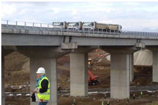
Fig. 1. Bridge of Transilvania Highway km 29+602,75 – km 29+801,25
