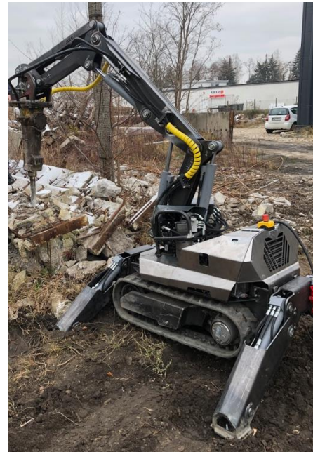
Fig. 3. Example of experimental testing during operation of construction robot
