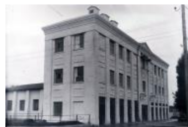
Figure 8. Building of power plant Ikervár (Fortepan 1928)
