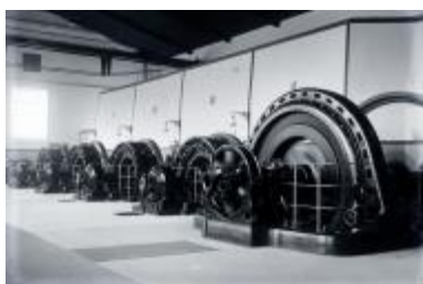
Figure 6. Engine house of power plant Ikervár (Fortepan 1928)
