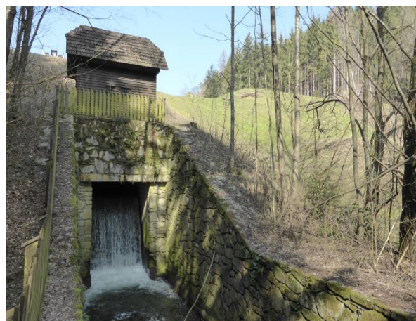
Photo 7 Flood control reservoir Prätisbach II. (by Günther Gruber 2014)
