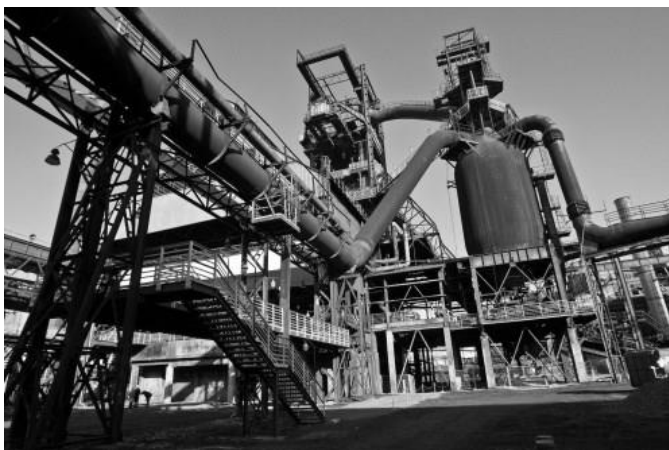
Figure 3 The Lower Area of Vítkovice
